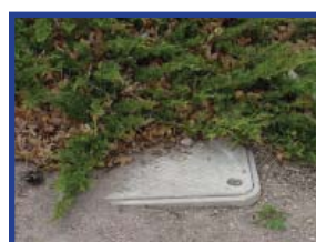
Inadequate clearance
