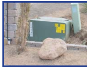
Inadequate clearance
