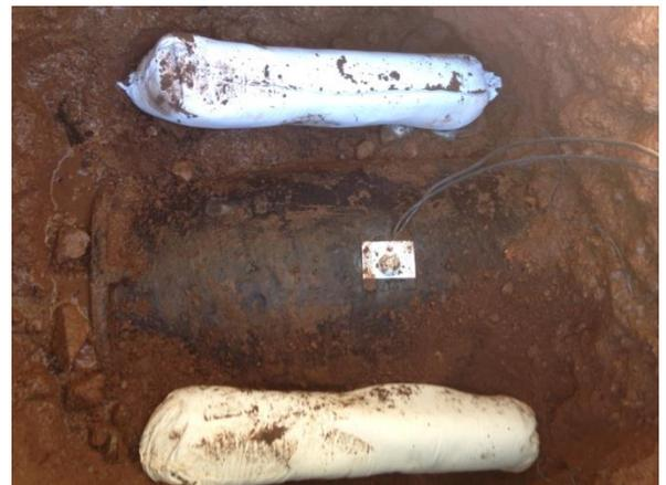
*Cathodic protection installed on a 20' water pipe.*
