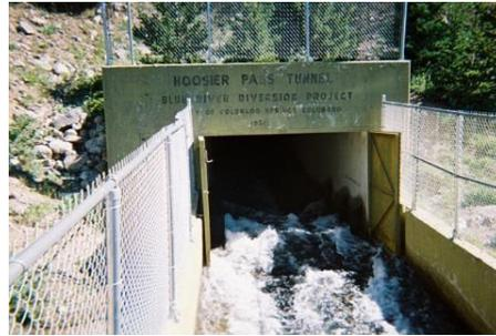
**Tunnel:** A below-ground channel used to transport water from other areas. Our tunnels move water through the Rocky Mountains.
