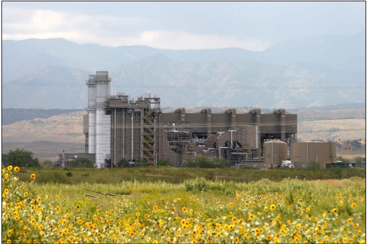
Figure A- 2: Front Range Power Plant
