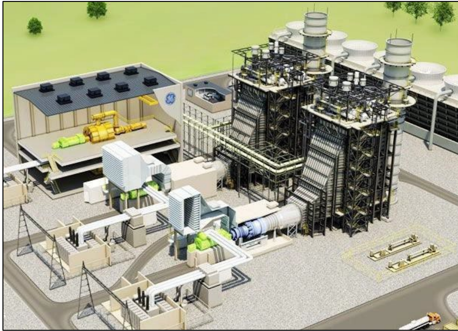
Figure C- 2: Combined Cycle Power Plant Layout
