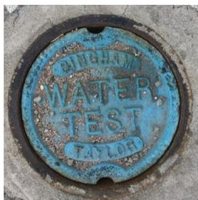
**General:** The Water CP Test Station offers the versatility of being buried in or near street pavement. Each 5.25-inch lid shall be painted “Blue” and shall have “Water Test” cast into the Heavy Duty H20 rated lid. The body shall be 15 inches in height and made of high impact plastic. A 5-terminal test board shall be attached to the lid. This test box will be used in conjunction with Cathodic Protection Test points and systems.
