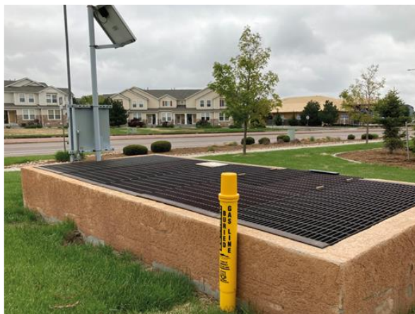
Natural gas regulator station.
