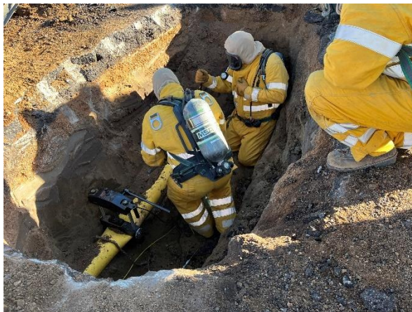
Gas construction crew repairing a gas leak. Photo credit, Jane Zook.
