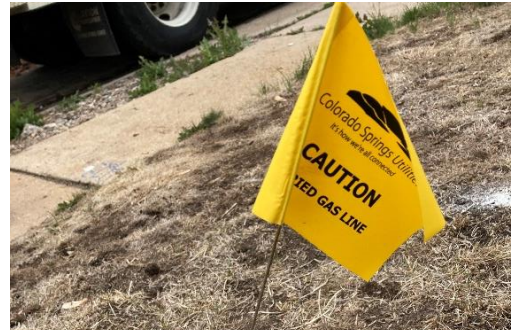
Yellow flag marking a buried natural gas line.
