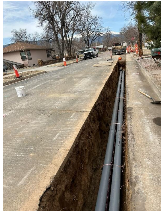
Electric project to underground sub transmission line in a weather vulnerable area along Nevada Ave.
