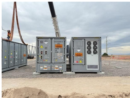
Lithium-ion batteries installed at the Jackson Fuller Substation in northeastern Colorado Springs.
