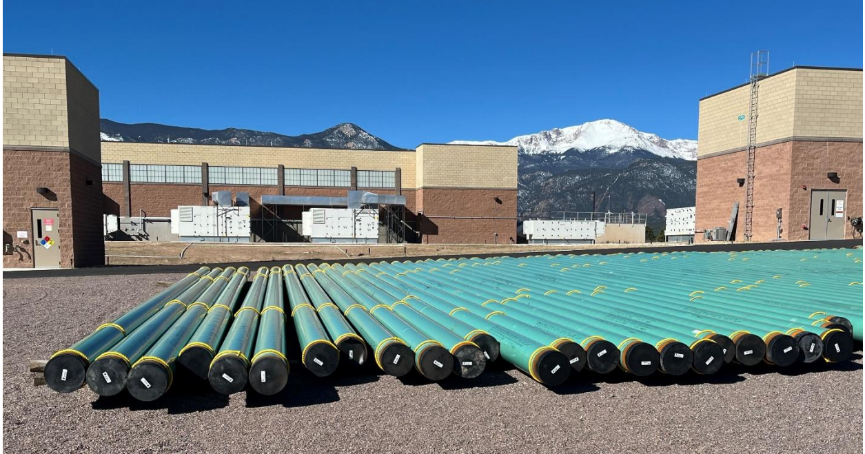
Gas pipeline main in preparation for a large-scale main replacement project.
