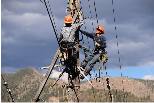
Linemen repairing a distribution line after a storm.
