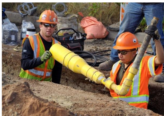
Natural gas construction crews installing pipeline.
