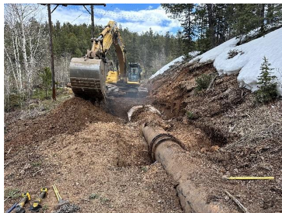
Pipeline removal at South Catamount Reservoir.
