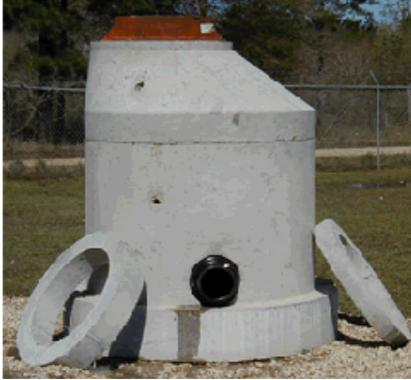
**General.** All Manholes shall have a minimum 4" wall thickness, consist of a base, barrel section and cone with ring and lid. Barrel sections and adjustment rings may be added as needed. See Detail Drawing [C3-1](#).
