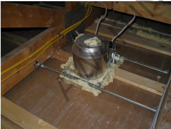
Air sealing is discovering all the nooks and crannies that allow air to leak in and out of the home and sealing them up! Gaps and open seams can form along the edges of doors and windows and even around the can lights in your ceiling.
