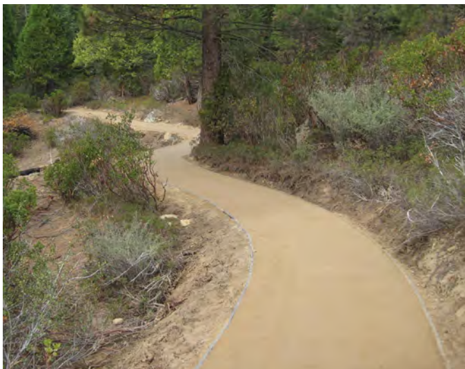
Figure 2–18. A trail that complies with trail accessibility guidelines with firm and uniform tread. Sequoia National Forest, California. USDA photo by Scott Johnson.
