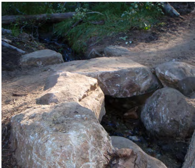
Figure 4–15. Rock culvert on the Lake Tahoe Basin Management Unit, California. USDA photo by Garrett Villanueva.
