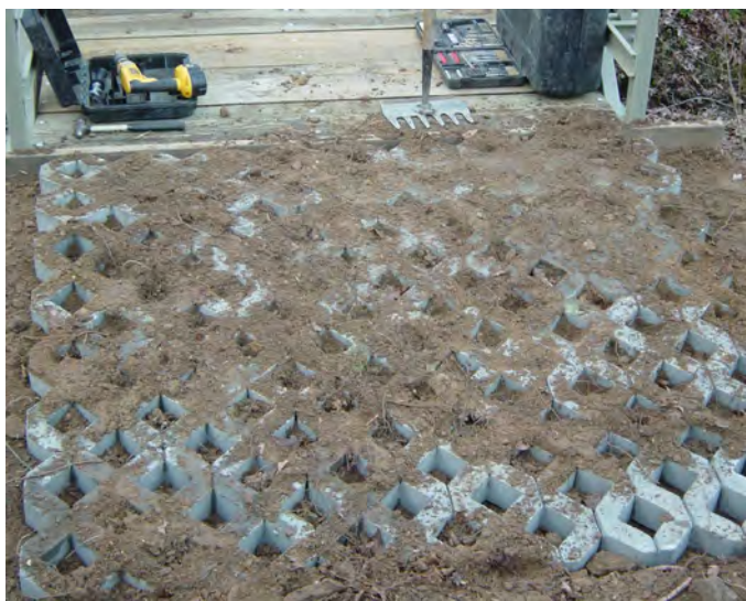
Figure 4–24. Concrete pavers are good for hardening trail structure approaches on trails designed for motorized use. The voids need to be filled with gravel, sand, or native soil and compacted. Sam Houston National Forest, Texas. USDA photo.
