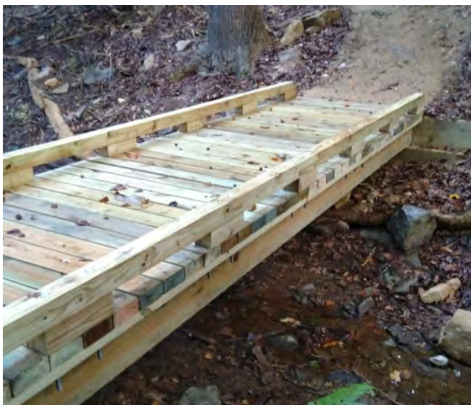
Figure 4–26. Example of curbing made of dimensional lumber with bull rail and scupper blocks. Greenbrier State Park, Maryland. Maryland Department of Transportation photo by Cheryl Ladota.
