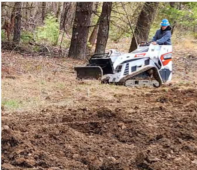
Figure 7–16. Stand-on skid steers being used on the George Washington and Jefferson National Forests, Virginia. USDA photo by Scott Johnson.
