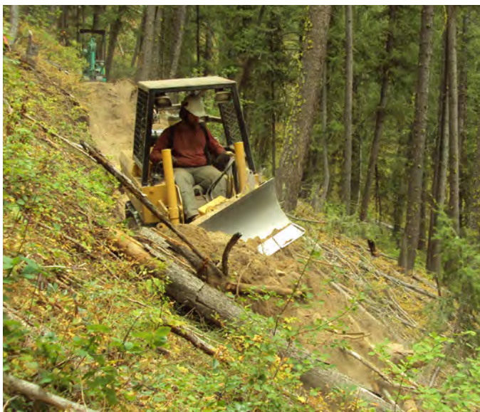
Figure 7–15. A trail-size dozer. Boise National Forest, Idaho. USDA photo by Scott Johnson.
