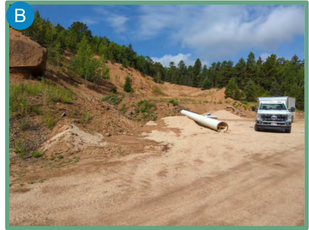
Figure 3: Construction Staging Area Along Catamount Shortcut Road
