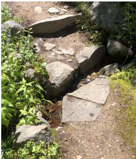
Figure 4–18. Open-top drains can be made of rock or wood. Pike–San Isabel National Forests, Colorado. USDA photo by Adam Carroll.
