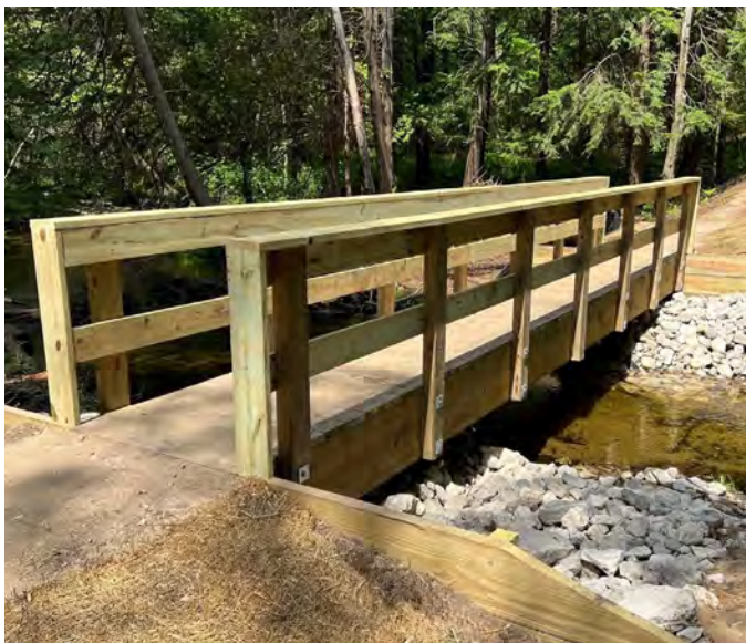
Figure 4–27. Trail bridge railing system with posts and top and intermediate rails. Huron–Manistee National Forests, Michigan. USDA photo.
