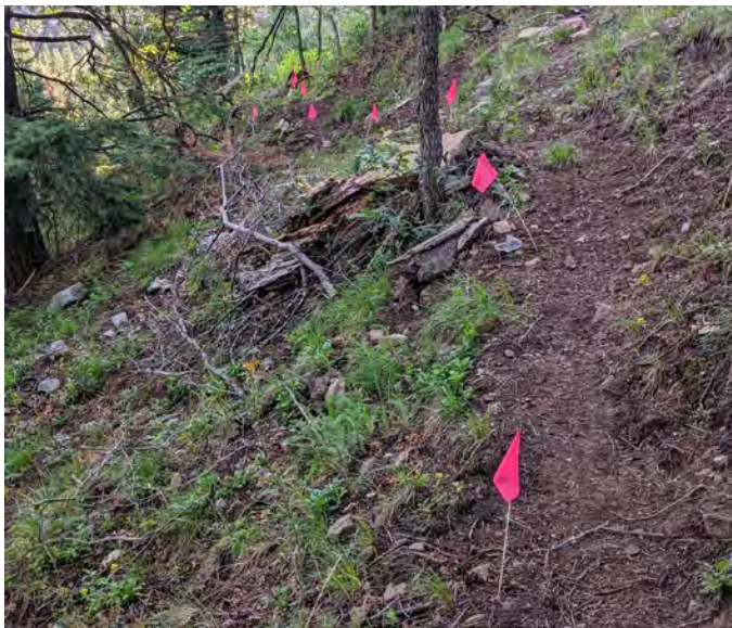
Figure 6–6. Pin flags mark the exact location of the trail tread and give you a good feel for the flow of the trail. Cibola National Forest, New Mexico. Courtesy photo by Jenny Blackmore.
