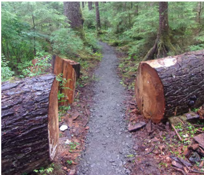
Figure 3–9. Cut logs help to keep the trail in place and the proper width. Refer to the TMO for trail design specifications, including appropriate trail width. Tongass National Forest, Alaska. USDA photo by Laurent Deviche.
