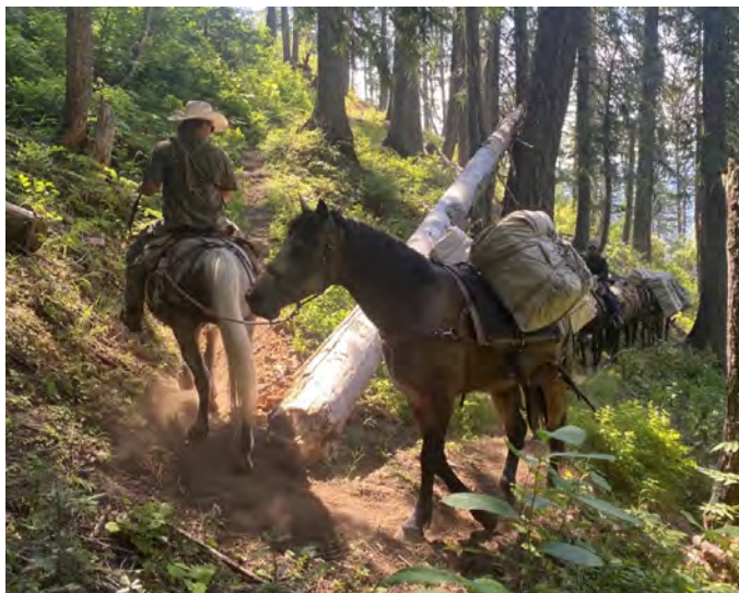
Figure 4–34. Pack stock navigate around a guide structure on a modified climbing turn. Nez Perce–Clearwater National Forests, Idaho. USDA photo by Ella Bradley.
