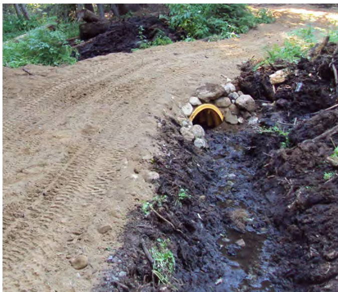
Figure 4–16. Arch culverts are a good option for moving water under a trail while keeping a natural stream bottom. Boise National Forest, Idaho. USDA photo by Scott Johnson.
