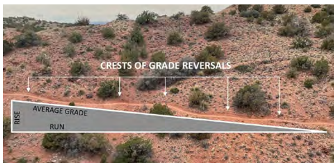
Figure 6-7. Grade reversals are much more effective than constructed drainage features. Grade reversals in this image are where the trail rises and falls. Water from the slope above will run off the trail in these areas instead of down the trail. Cibola National Forest, New Mexico. USDA photo by Kerry Wood.
