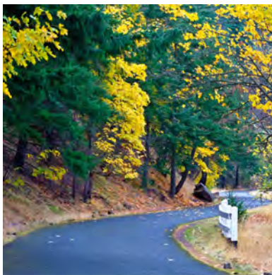
Figure 2–17. A fully developed (class 5) trail has a firm and uniform tread, less than a 5–percent grade, and likely meets accessibility guidelines. Columbia River Gorge National Scenic Area, Oregon. USDA photo.
