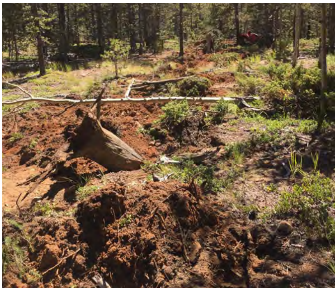
Figure 6–16. Completely block off abandoned trails. Plant native grasses and shrubs or place deadfall and other large debris to fill the opening left by the abandoned trail. Pike-San Isabel National Forests, Colorado. USDA photo by Scott Johnson.
