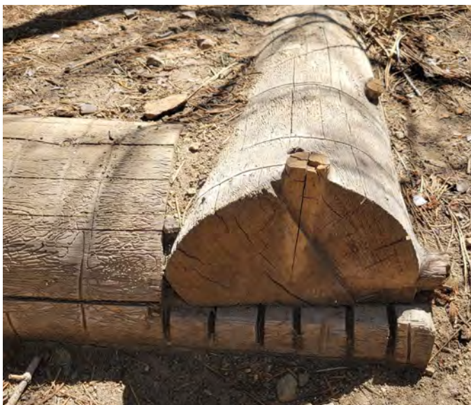
Figure 4–43. An example of a square notch on timber steps. Inyo National Forest, California. USDA photo by Jess May.
