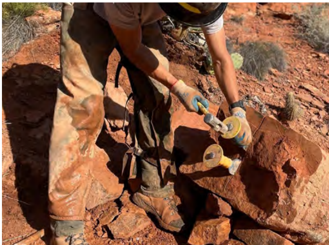
Figure 4–38. Shaping rock with rock chisels. Coconino National Forest, Arizona. USDA photo by Kevin Kuhl.
