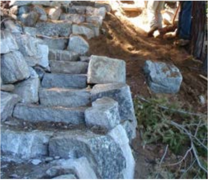
Figure 4–47. Installing overlapping rock steps with side retainer rocks. Lake Tahoe Basin Management Unit, California. USDA photo by Garrett Villanueva.
