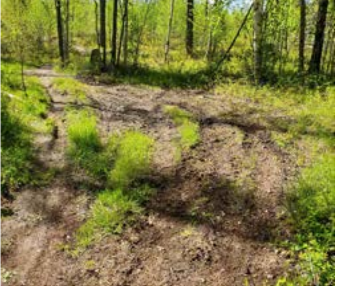
Figure 6–15. A candidate trail for a causeway structure or decommissioning and rerouting. Flathead National Forest, Montana. USDA photo by Jess May.
