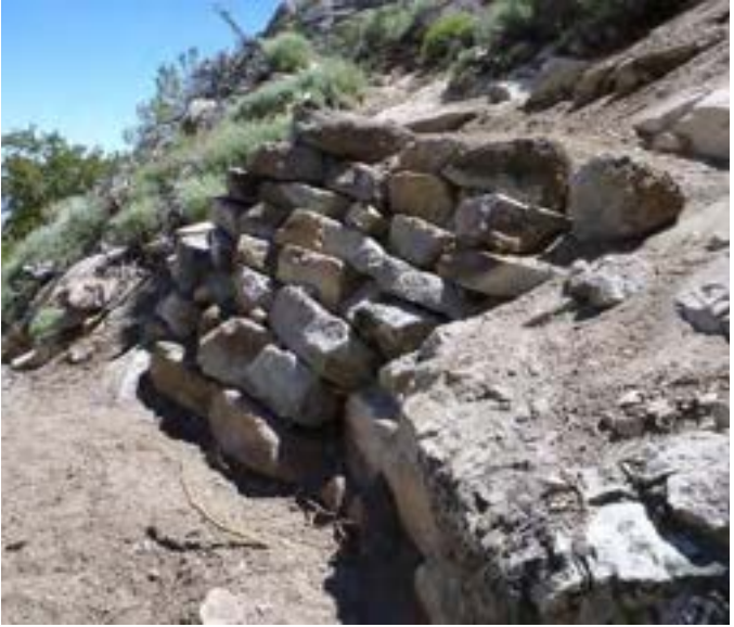
Figure 4–36. A rock retaining wall can be used to support the trail tread or hold back the backslope. Inyo National Forest, California. USDA photo by Jess May.
