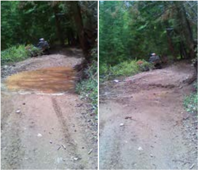
Figure 4–6. Installing knicks into existing trails will drain puddles from flat areas. This knick will require frequent maintenance because it's draining to the outside of a curve in the trail. Fishlake National Forest, Utah. USDA photos by Nathan Conder.
