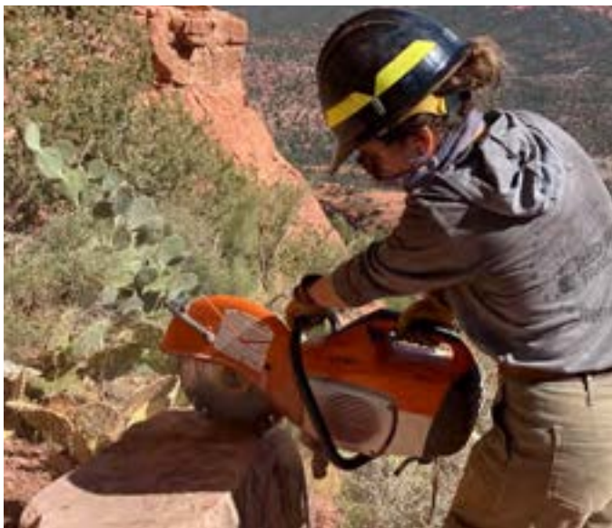
Figure 4–49. Cutting rock with a gas-powered rock saw. Coconino National Forest, Arizona. USDA photo by Kevin Kuhl.
