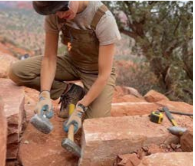
Figure 4-48. Splitting rock with a stone sledge. Coconino National Forest, Arizona. USDA photo by Kevin Kuhl.
