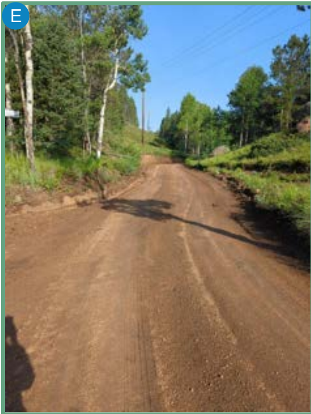
Figure 8: Colorado Springs Utilities Service Road
