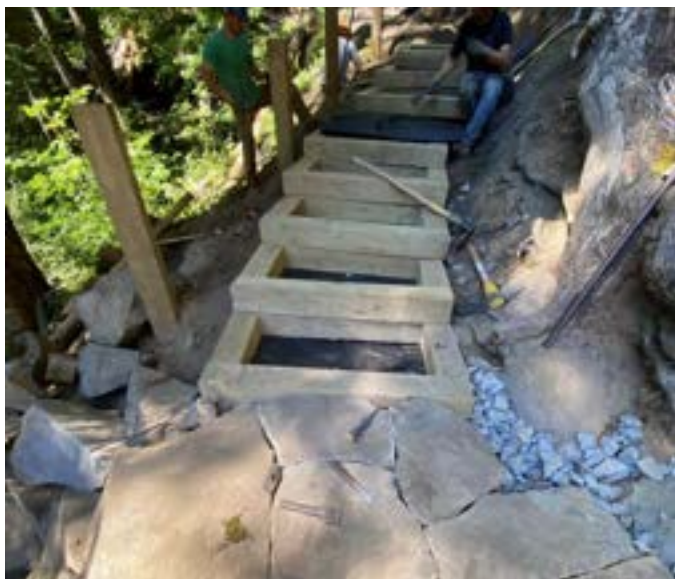
Figure 4–54. Overlapping timber steps being constructed on a hiking trail. The steps will be filled with crushed rock and overlain with fill material. Willamette National Forest, Oregon. USDA photo by Christopher Beitner.
