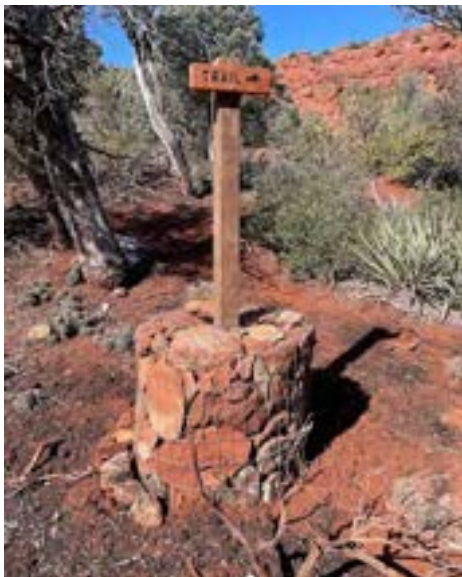
Figure 5–5. Gabion foundation for a signpost. Coconino National Forest, Arizona. USDA photo by Kerry Wood.
