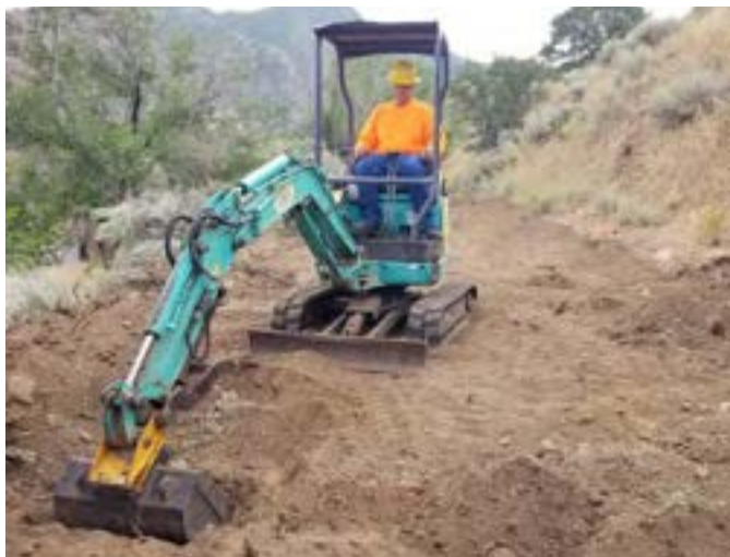
Figure 7–14. A mini excavator. Weber Basin Job Corps, Utah. USDA photo by Scott Johnson.
