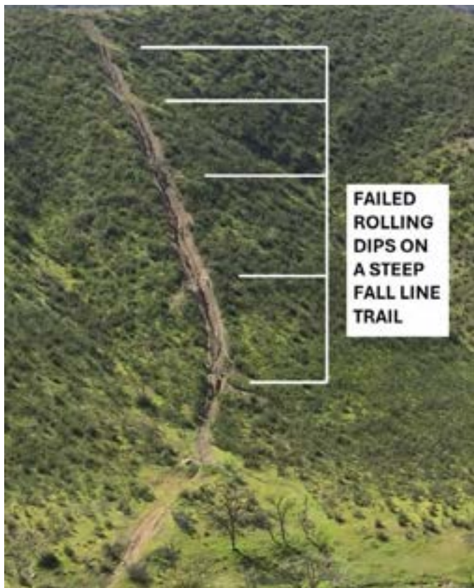
Figure 2-23. Heavily eroded fall line trail with several failed rolling dips. Mendocino National Forest, California. USDA photo by Scott Johnson.
