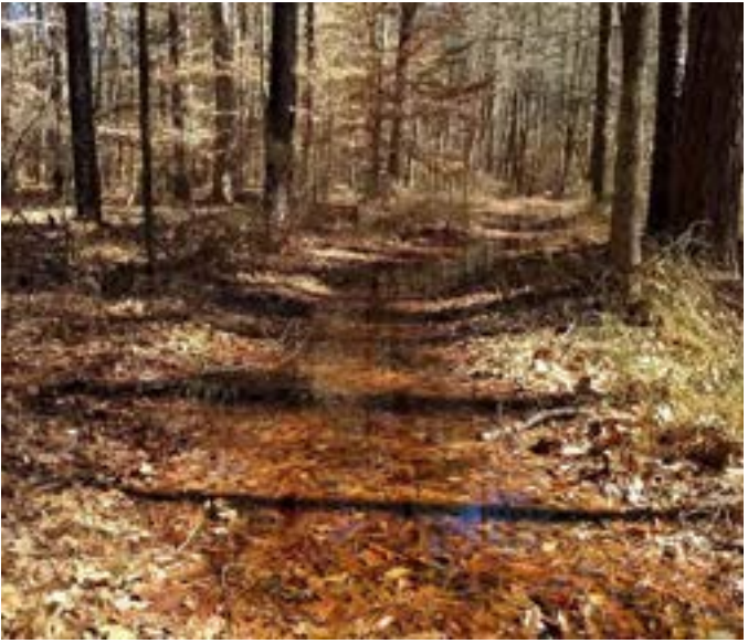
Figure 4–8. Standing water results in soft, boggy tread. Water is pooling in this flat trail segment. Ideally, the trail would be relocated onto the slope uphill. However, if relocation is not possible, the trail manager could install a drainage structure. Baltimore, Maryland. Maryland Department of Transportation photo by Cheryl Ladota.
