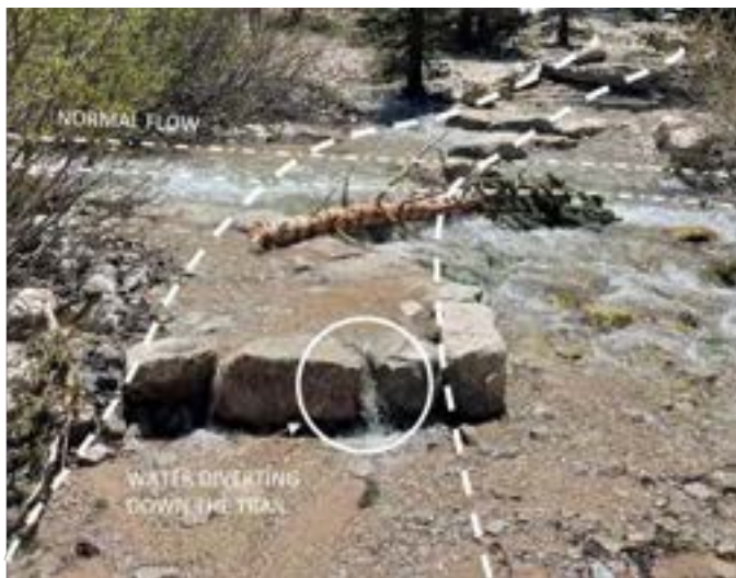
Figure 3–18. Stream at flood stage diverting down a trail that is approaching from a lower angle. Inyo National Forest, California. USDA photo by Jennie Leonard.
