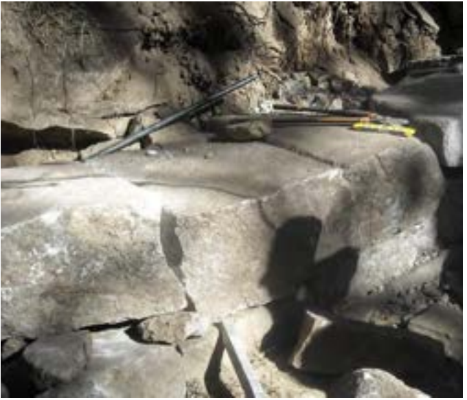
Figure 4-37. Rock wall foundation using quarried and cut rock. Lake Tahoe Basin Management Unit, California. USDA photo by Garrett Villanueva.
