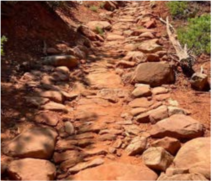
Figure 4-55. Rocks can be used to armor sections of heavily used trail. Coconino National Forest, Arizona. USDA photo by Kevin Kuhl.
