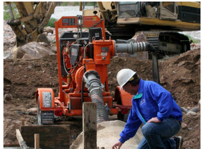
Water construction employee works on a creek crossing.
