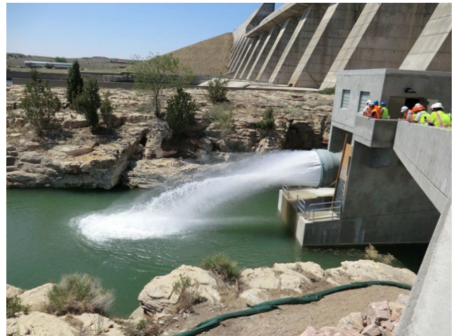
SDS Pueblo Dam connection test, 2012.
