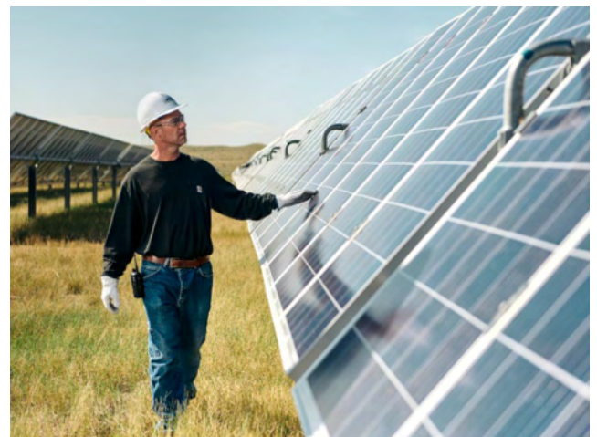
Employee with solar panels at the Pike Solar Array.
