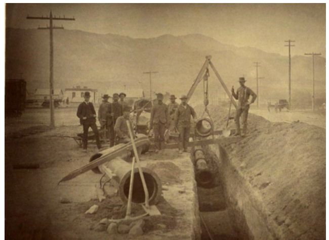
Water construction workers laying a pipe segment.
