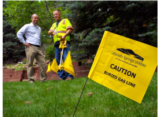
Yellow flag marking a buried natural gas line.
