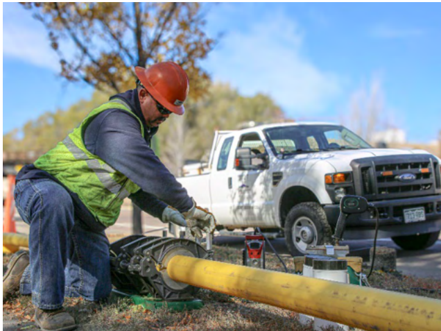
Natural gas employee working on a pipeline.
