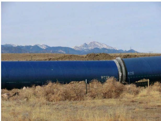
Southern Delivery System pipeline.
