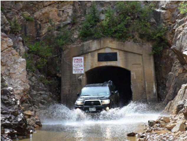
Vehicle exiting the Twin Lakes Tunnel.
