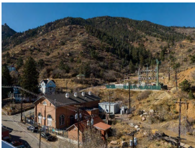
Manitou Springs Hydroelectric Plant.
