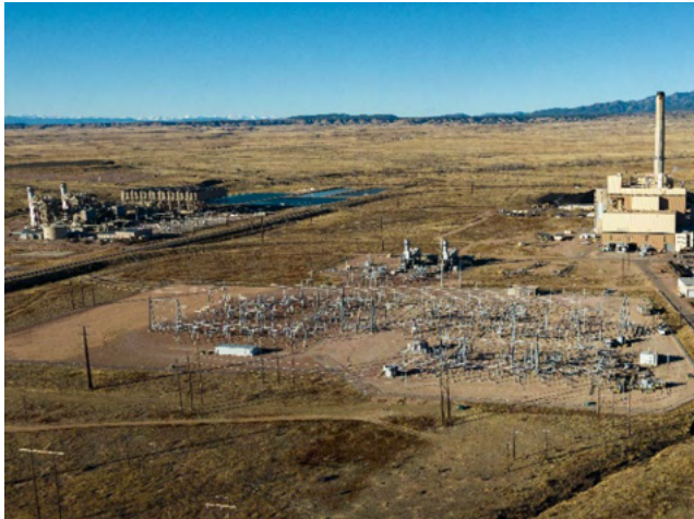
Front Range Power Plant (left) and Nixon Power Plant (right) on the Clear Spring Ranch property.
