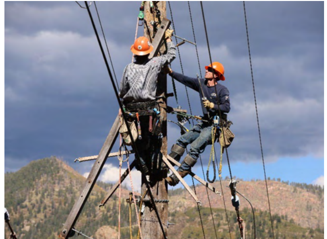
Linemen repairing a distribution line after a storm.
