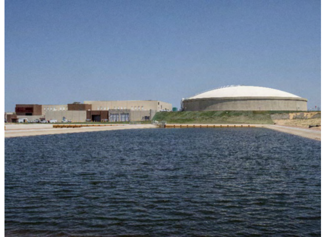
Edward W. Bailey Water Treatment Plant.
