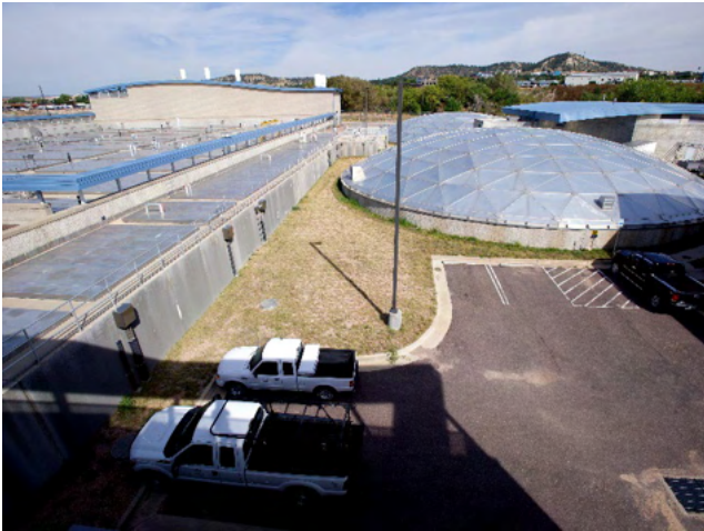
J.D. Phillips Water Resource Recovery Facility.
