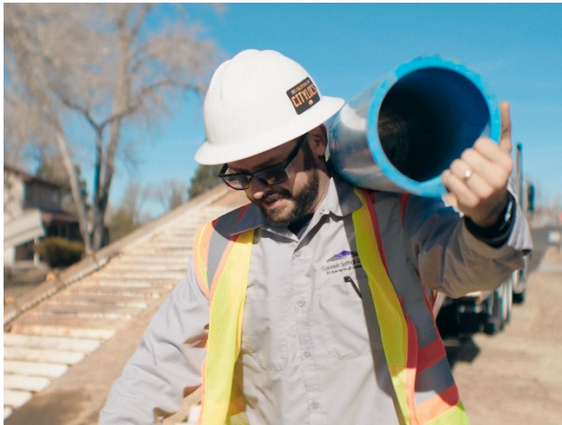
Water employee carrying a section of pipeline.
