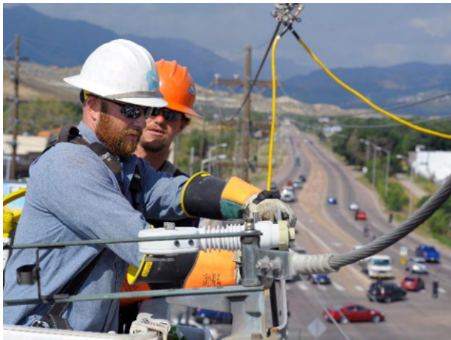
Electric employees working on a power line.
