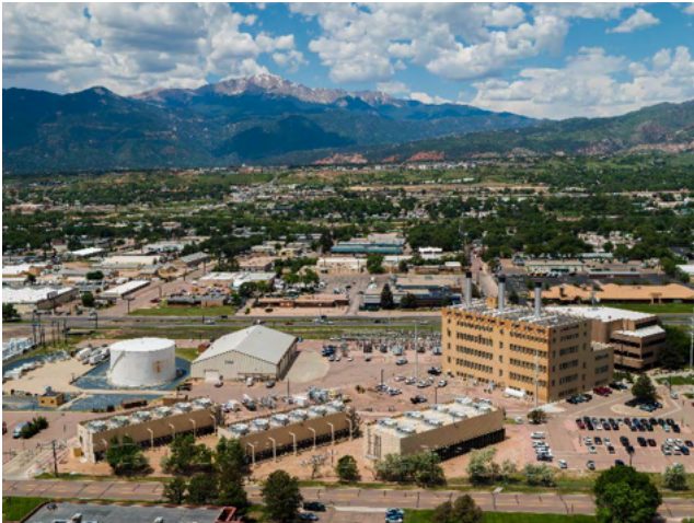
Birdsall Power Plant.
