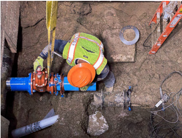
Water construction crew installing a new valve in the water distribution system.
