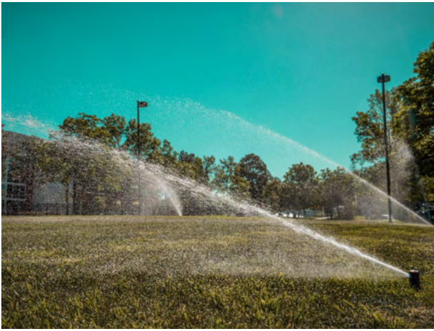
Sprinkler system watering a commercial lawn.
