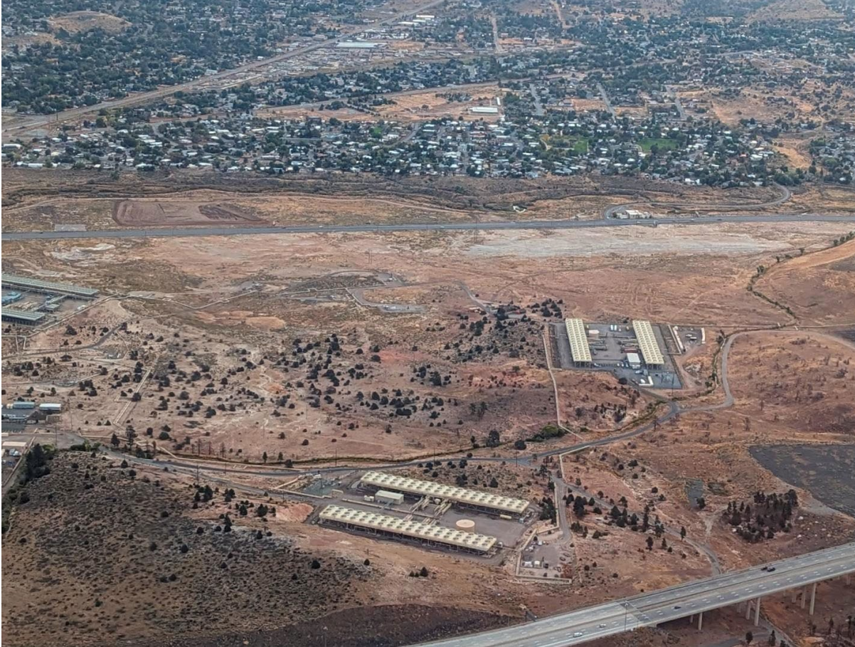
Ormat Steamboat Hills Geothermal Power Plant in Reno, Nevada. Photo by Bryce Carter. October 2023.
